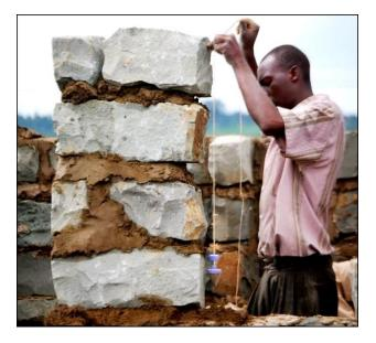
With this in mind Amos introduces the idea of the "plumb line". Now a plumb line is a tool consisting of a small, heavy object attached to a string or rope. It is used to see if something such as a wall is perfectly vertical. In other words, a plumb line measures if something is true or not.
